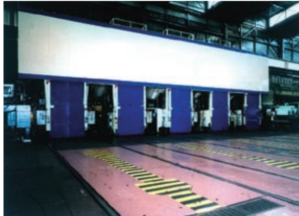
Fully continuous cold strip mill
